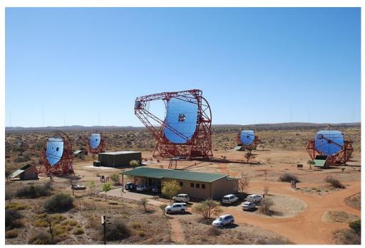
The fifths telescope H.E.S.S II is situated in the diagonal cross hair of the square and has a mirror made up of 875 hexagonal mirror facets with 0.9m diameter. Together this amounts to 614 m<sup>2</sup> or a mirror of 28 m diameter! The overall height of the structure is 40 m and the overall weight 600 tons. It is currently by far the largest reflective telescope in the world.
